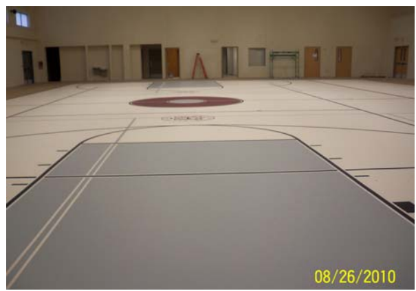
The gym floor is almost done!!
